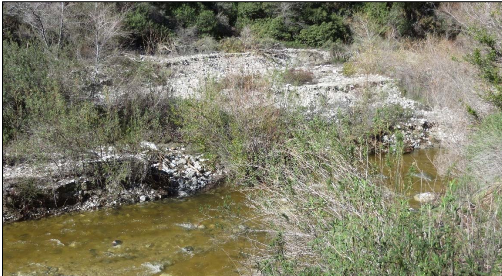
Figure 3-10. Multiple levels of flood deposits confining the active channel of the Arroyo Seco, about 5,500 feet upstream of Brown Mountain Dam.
