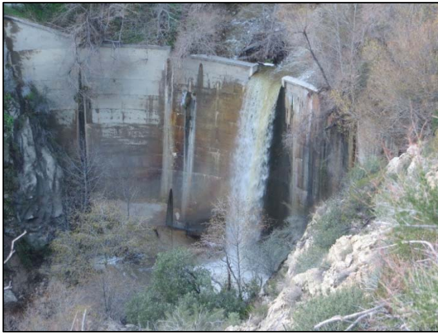
a. View of water flowing over spillway
