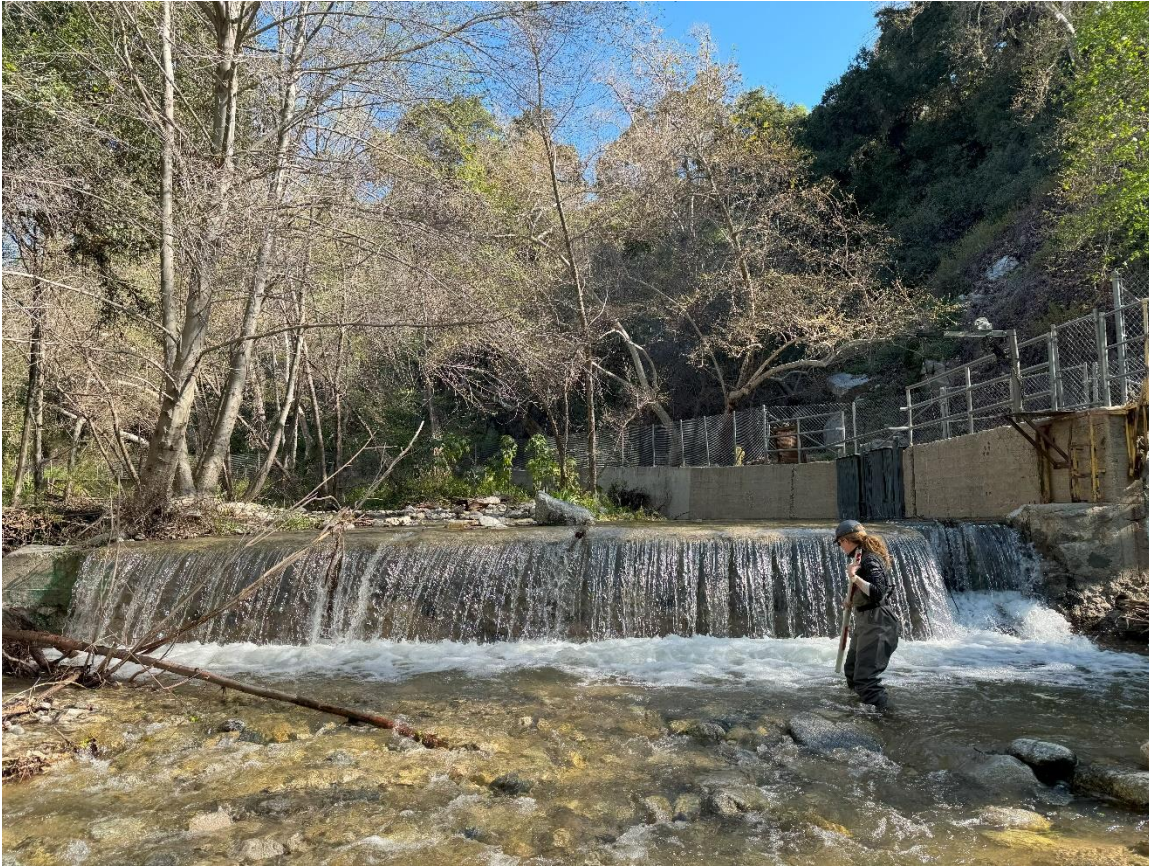
Figure 6. Pasadena Water and Power diversion weir at river mile 1.81.
