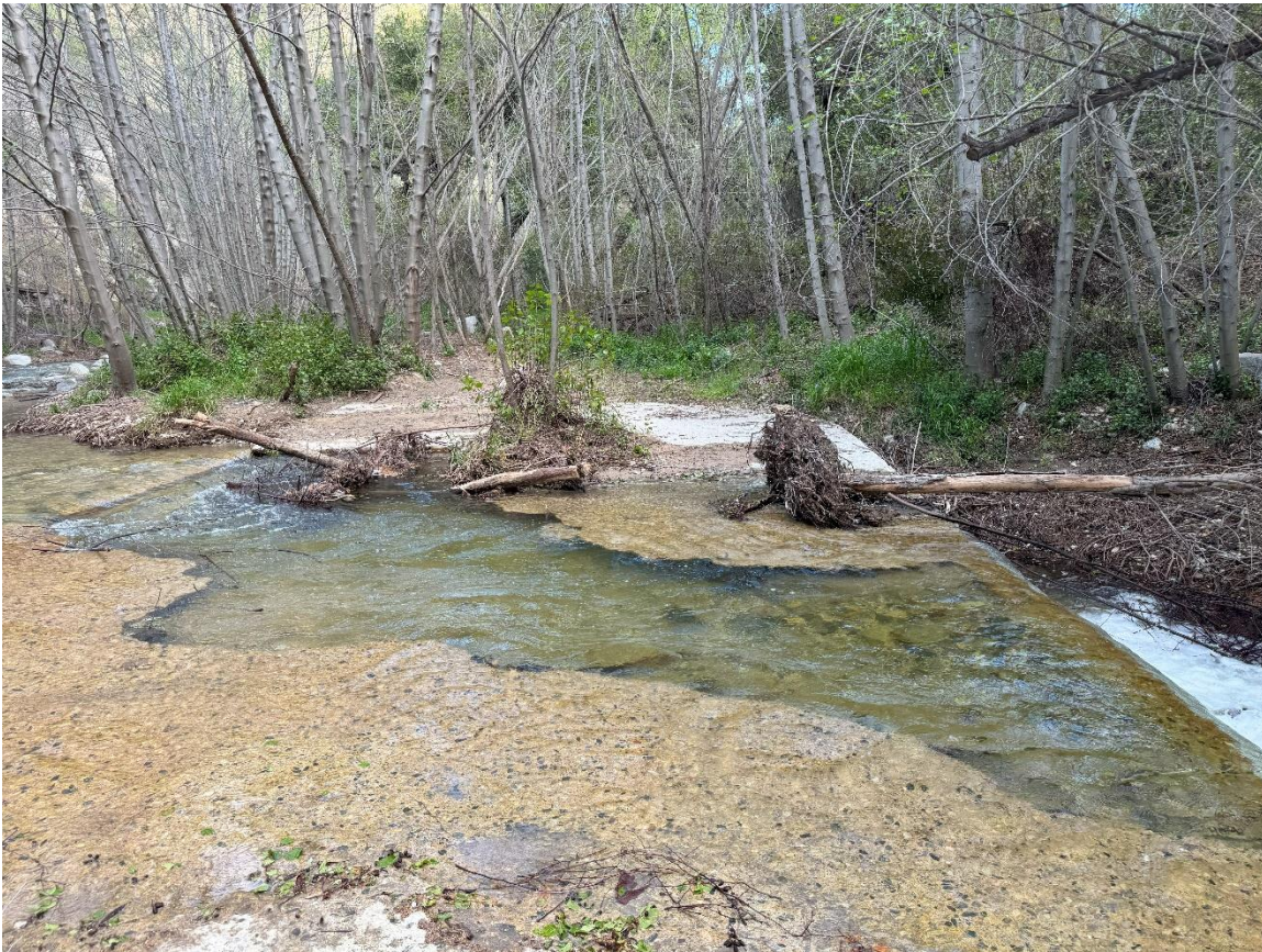
Figure 11. Arizona crossing at river mile 4.23.
