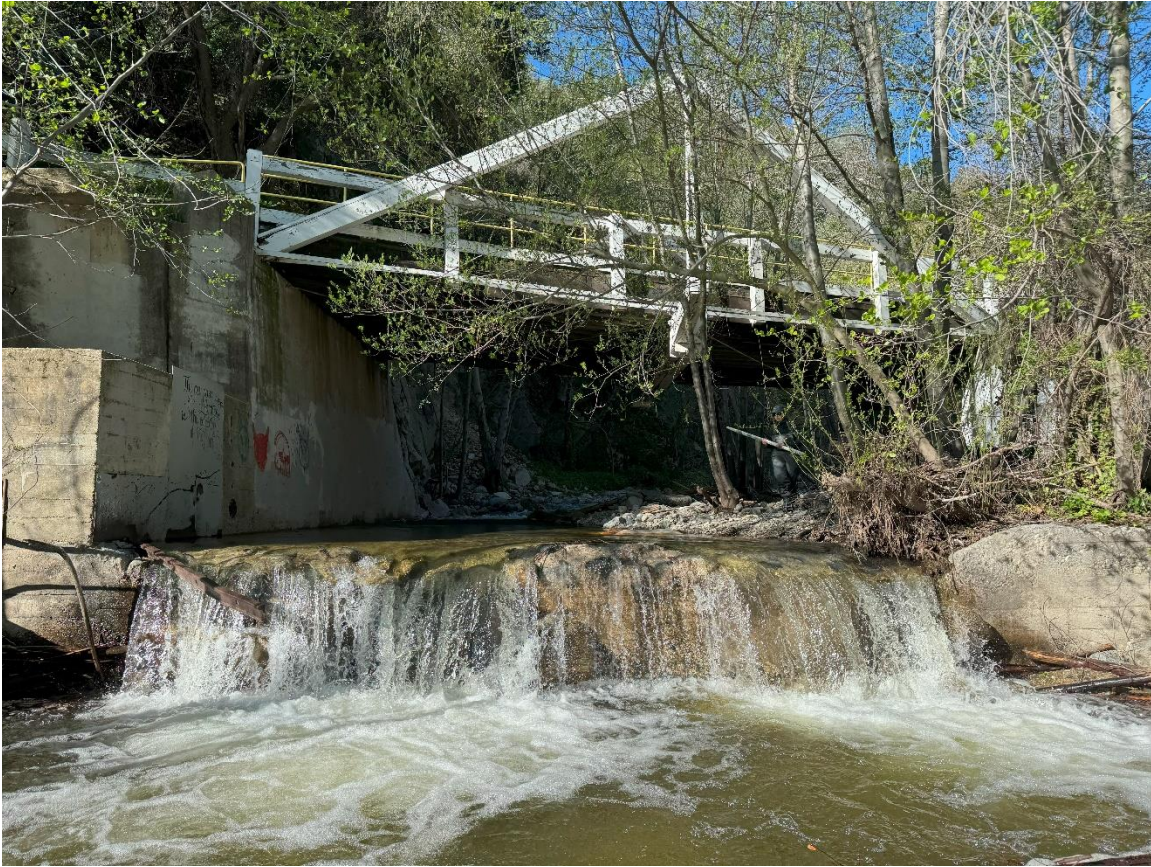
Figure 5. First crossing at river mile 1.71.
