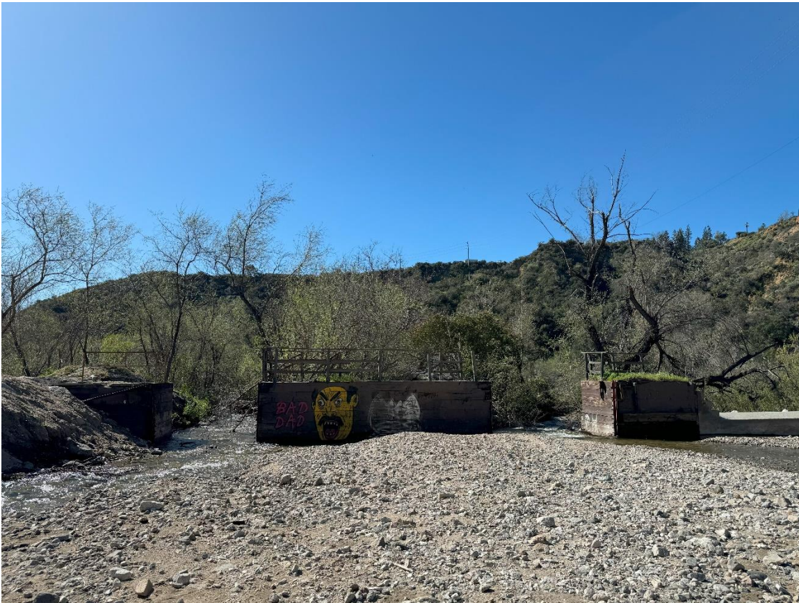
Figure 7. Sediment headworks at river mile 2.19.
