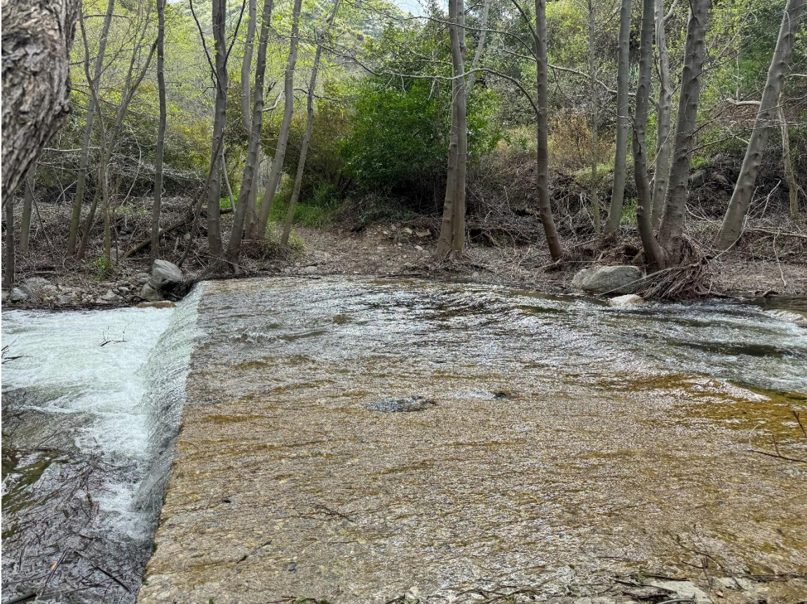
Figure 15. Arizona crossing at river mile 5.19.
