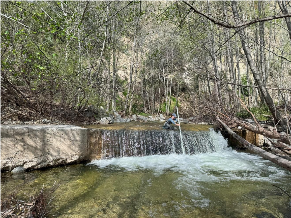
Figure 14. Arizona crossing at river mile 4.91.
