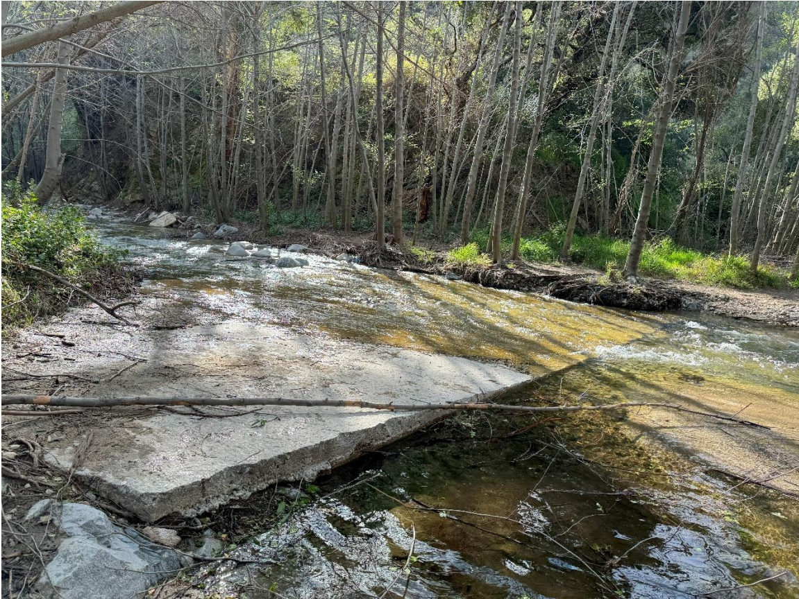
Figure 12. Arizona crossing at river mile 4.30.
