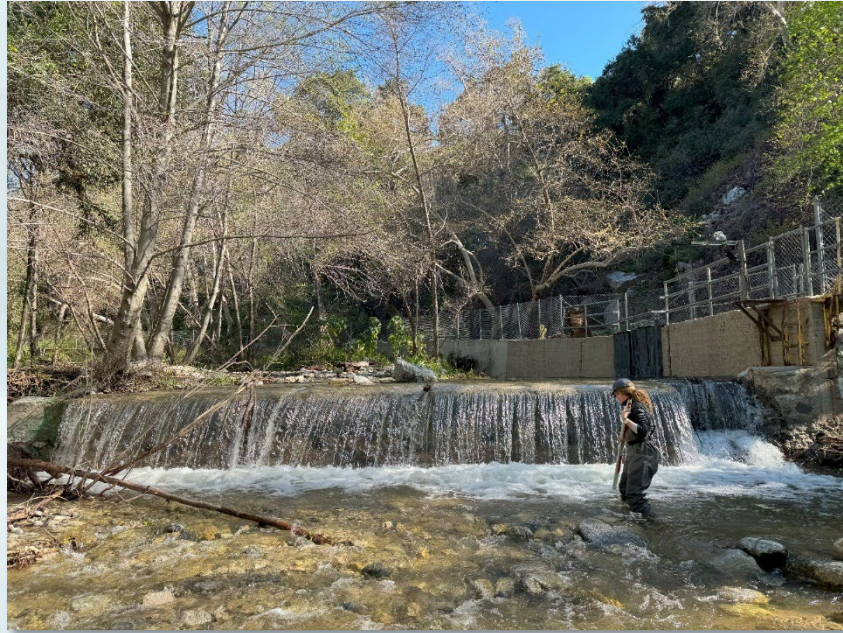
PWP Diversion (RM 1.81)
