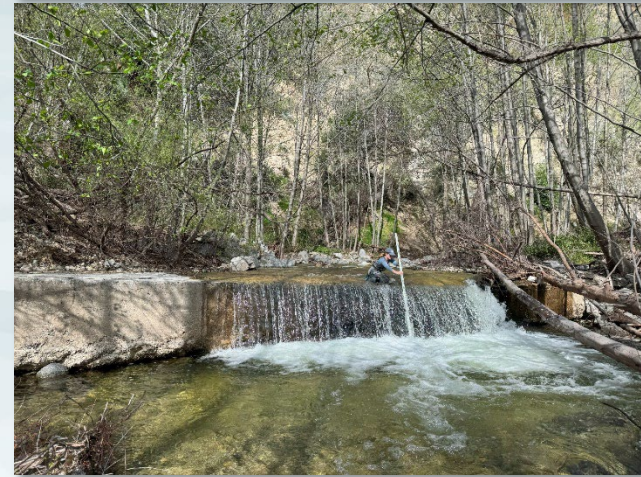
Arizona Crossing (RM 4.91)
